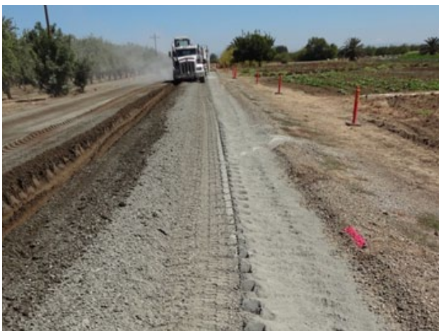
Figure 4. Type II Cement Was Applied to the Pulverized Existing Pavement Materials
