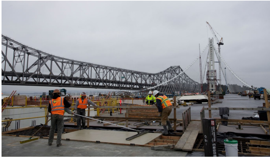
Figure 1. Placing fast-setting Concrete at Seismic Joints
