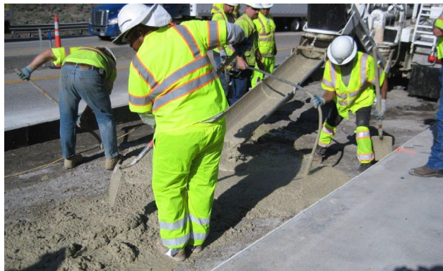
Figure 3. Placement of Rapid Set
