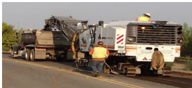
Figure 2. Cold milling of the Existing Pavement on Ord Ferry Road
