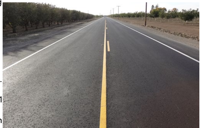
Figure 9. Completed Ord Ferry Road FDR-C Project with Cold Central Plant Recycling and HMA Overlay
