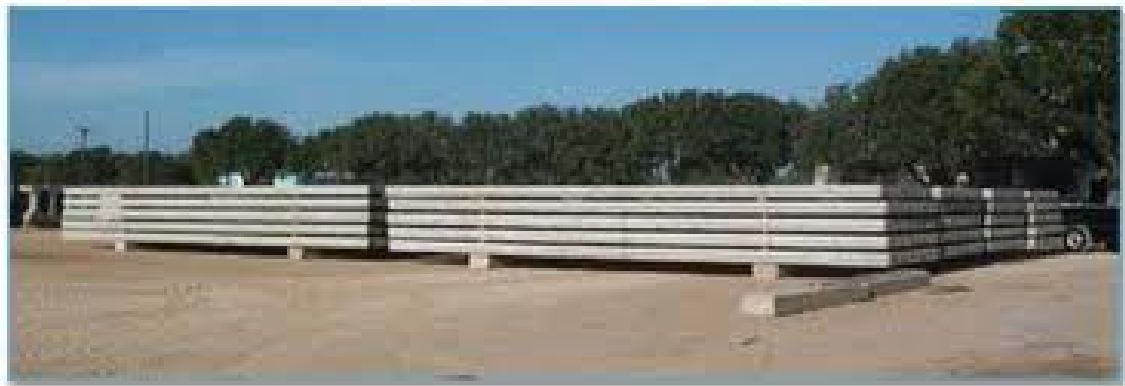
Figure 1. Innovations: Precast Concrete Pavement System (precast modular concrete panels at offsite location)
