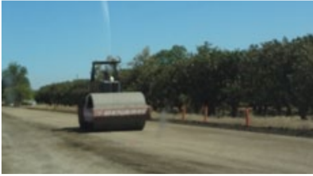
Figure 7. Roller Compactor to Finish the FDR-C Compaction
