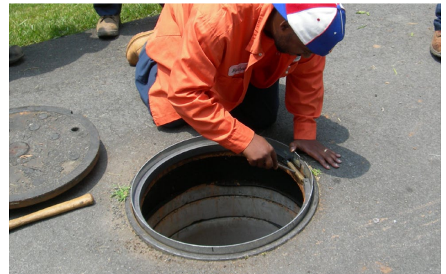
Figure 1. Installing Riser Ring onto Old Manhole Ring
