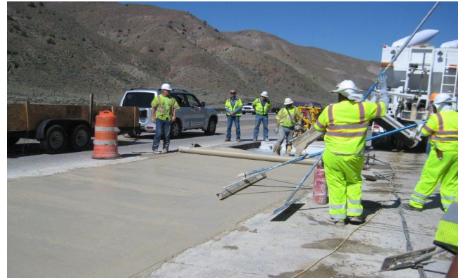
Figure 4. Finishing of Rapid Set
