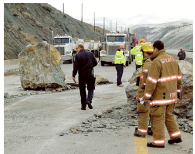
Figure 1. Damaged Slabs by Boulders
