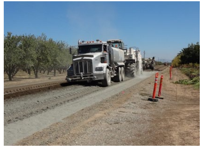
Figure 5. FDR Mixing Operation
