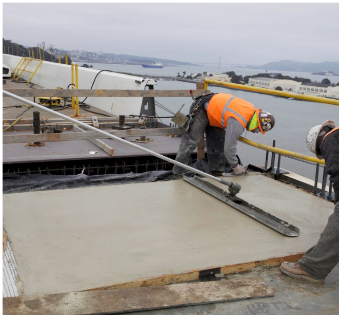
Figure 2. Hand Finishing Seismic Joint Areas
